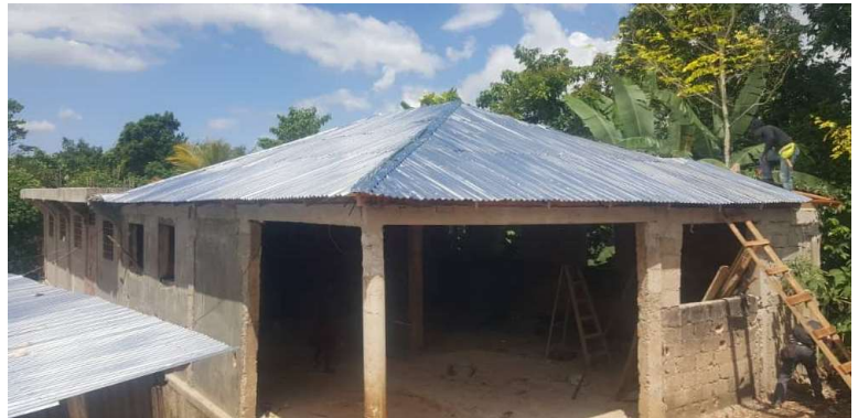
Second orphanage building during repair and construction completion
