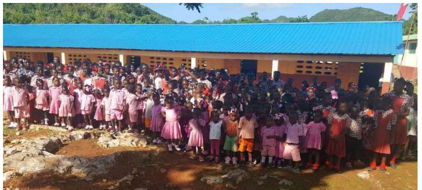
Elementary school building grades 1-6 with new roof
